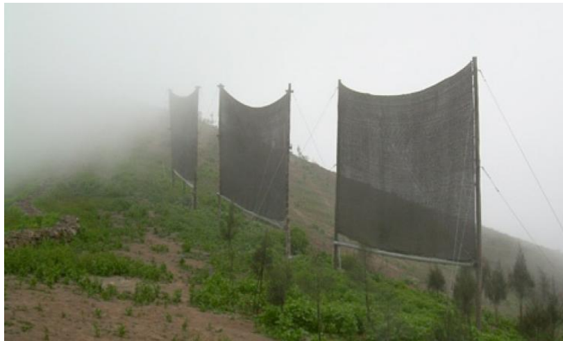
Figure 15. Large fog collectors installed in a foggy, mountainous area
